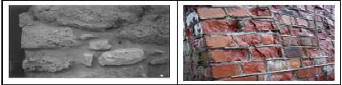
Fig: 2. Show the weakness of Components of the brick and mortars brick walls of the historical influence of long-term deterioration
