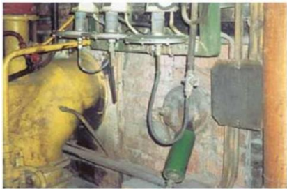
Fig. 1.2: Installation of an Acoustics-T device on a DKVr-10 boiler.
